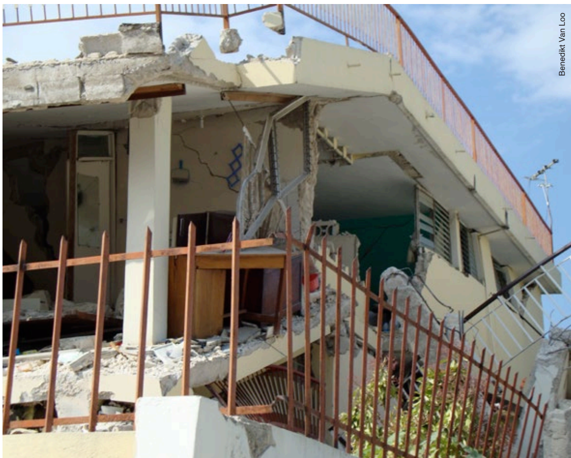
Destroyed buildings in Haiti following the 2010 earthquake.
